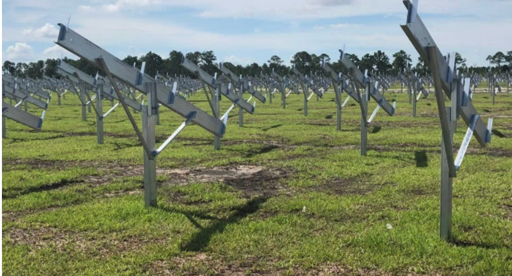
Figure 2-3 Proposed Solar Table Support Structures
